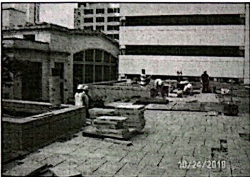
U.T. System – Ashbel Smith Hall Plaza Deck Waterproofing Replacement
