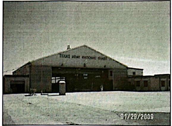
Martindale Army Air Support Facility San Antonio, Texas Metal Roof and Flat Roof Replacement Project
