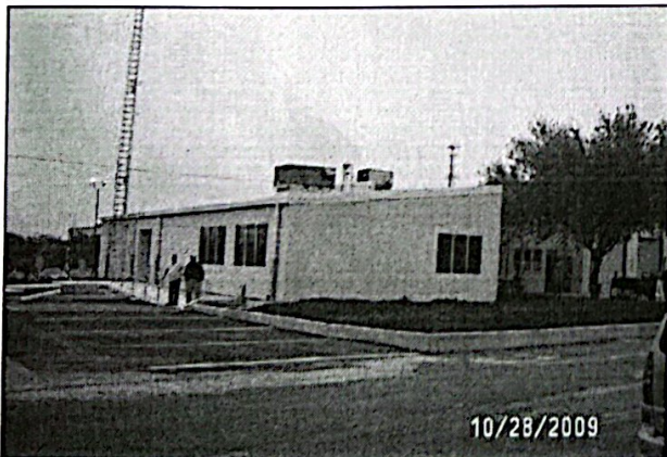
Bexar County Service Center Additions & Renovations San Antonio, Texas
