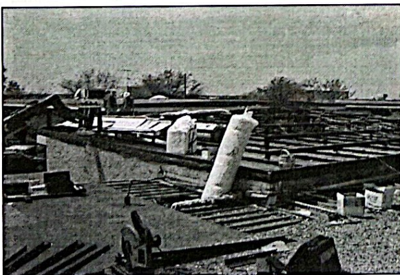
Medina Valley I.S.D. La Coste Campus Metal Roof Retrofit Project
